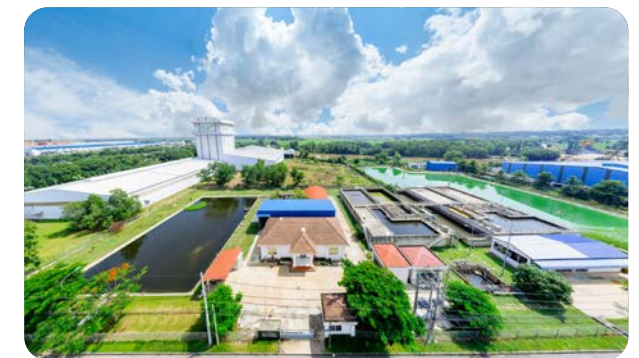
Wastewater treatment system for normal projects
