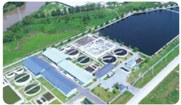
Wastewater treatment system for textile with dyeing projects • Design capacity: 65,000 m 3 /day.night • Current capacity: 12,000 m 3 /day.night
