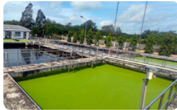
Wastewater treatment system
